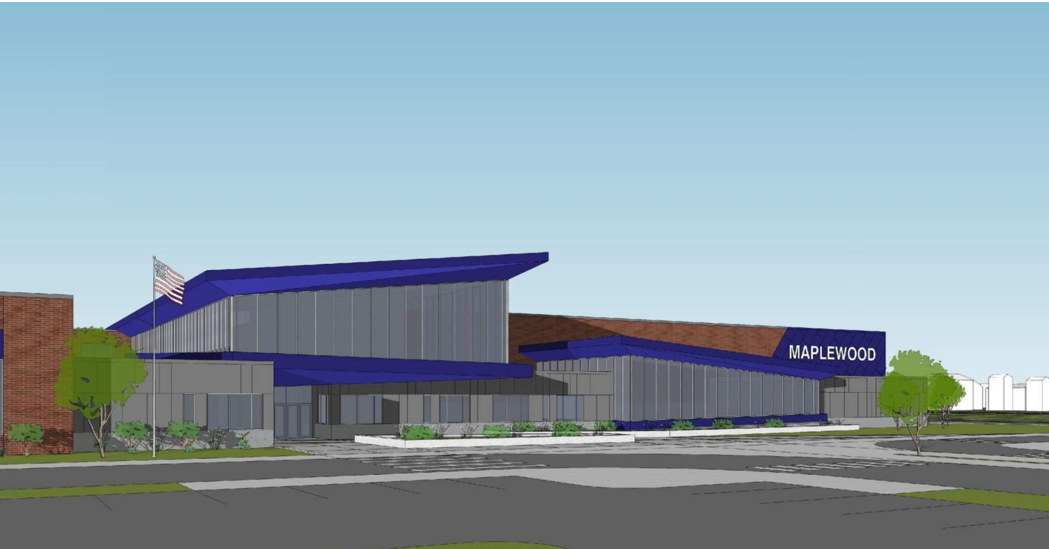
VIEW OF SOUTH ENTRY
